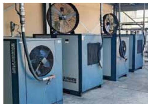
I compressori de La Padana presso la Speroni Water Pumps.
